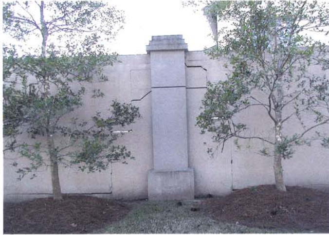
3rd Filing Wall - Perkins Road View
