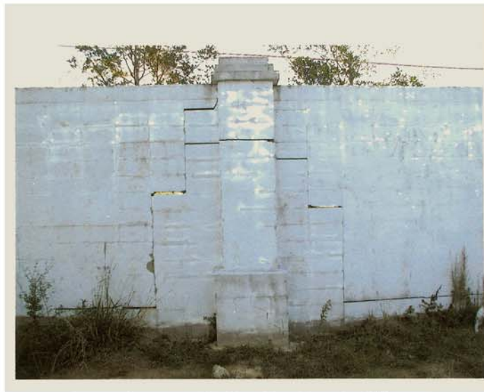
3rd Filing Wall - Backside View
