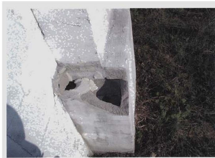
3rd Filing Wall Pilaster Footing - Backside View
